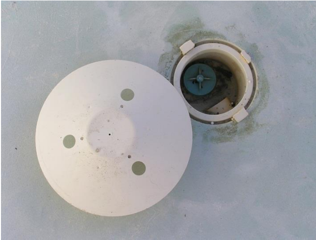
Fig 1 Typical main drain, with cover (removed) and hydrostatic valve top visible inside
