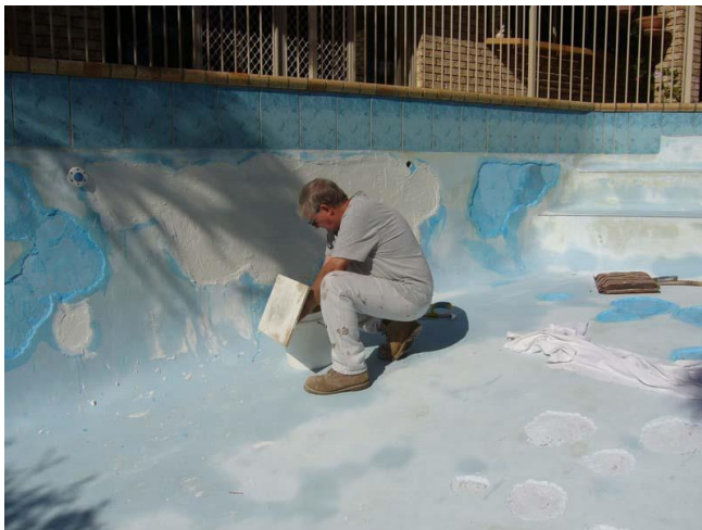
Undertaking repairs to Marcite, through to finished pool.
