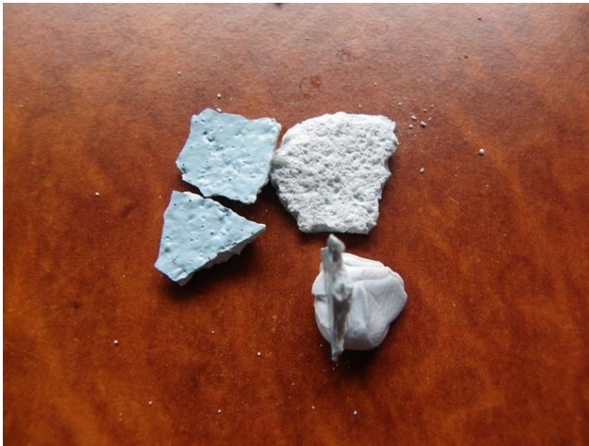
Pic 3. Showing underside of paint sample with, in this case Marcite attached. Here we see a weakness, basically a cohesive failure of the Marcite to the substrate. Bottom right sample is edge on, showing cross section.
