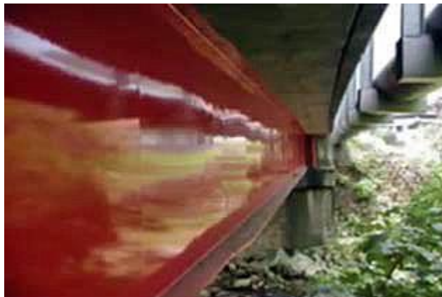
2016 after 23 years no signs of UV or any other damage (left)
