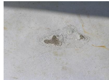
Typical surface issues with aged Pebble Tec and Marcite Pools from 5 years onwards
