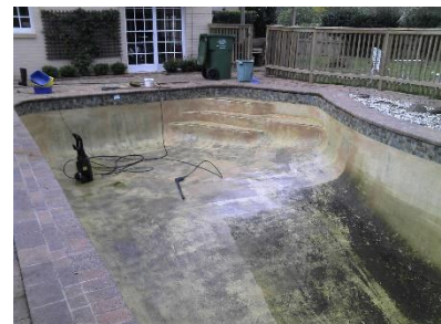
Typical surface issues with aged Pebble Tec and Marcite Pools from 5 years onwards
