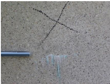
Typical surface issues with aged Pebble Tec and Marcite Pools from 5 years onwards
