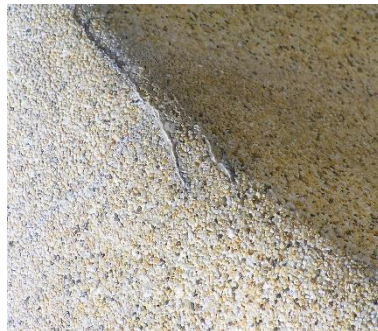
Typical surface issues with aged Pebble Tec and Marcite Pools from 5 years onwards
